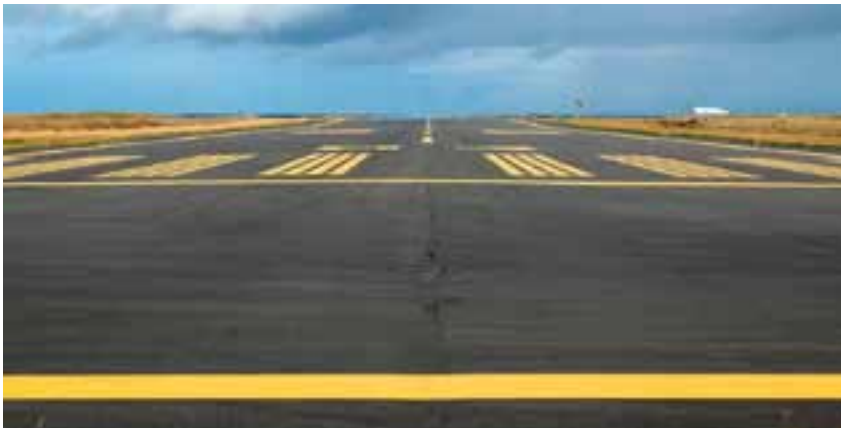
Runway with yellow markings in Norway. The Norwegian CAA have decided to ask Avinor to phase these markings out and to mark the runways white by 2017 at the latest 2 (Photo by Avinor)
